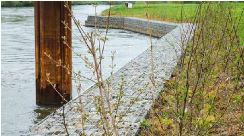
FLOOD PROTECTION RAWE-STONE BOXES WITH INTEGRATED NON PERMEABLE MAT WITH:
