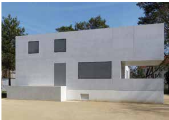
New Masters' Houses in Dessau; Architecture: Bruno Fioretti Marquez Architects; performance: Arbeitsgemeinschaft Betonlasur Berlin
