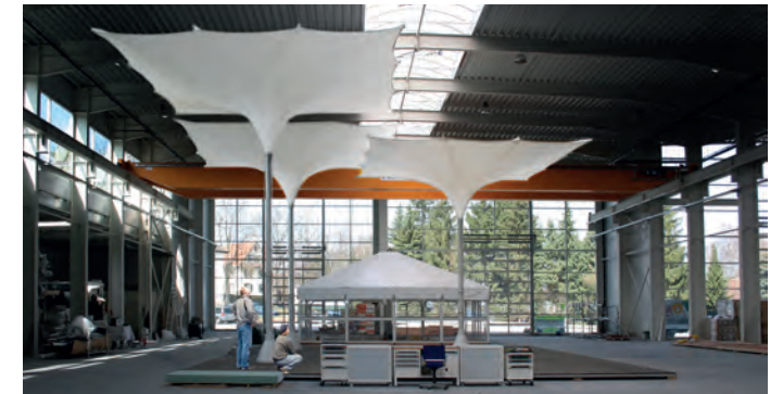
Final assembly with 30m span Wire
