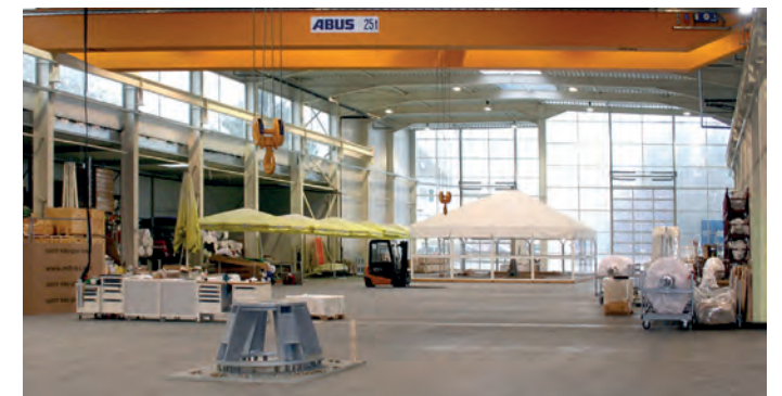
2x25 to overhead cranes
