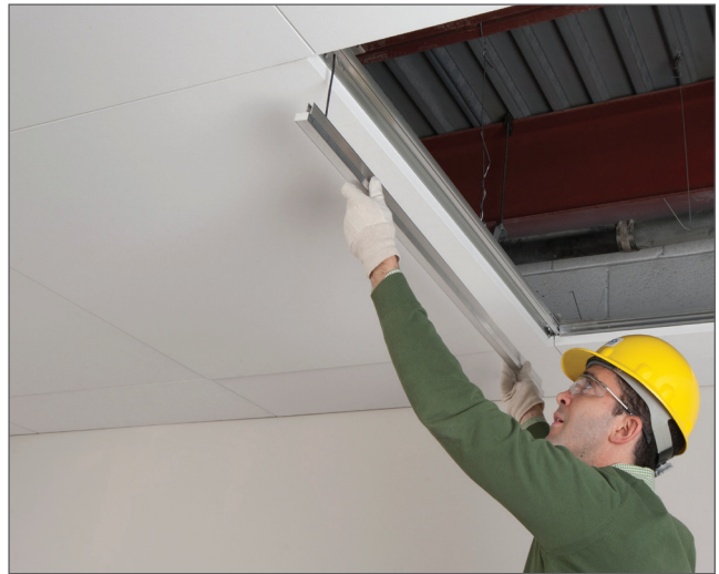
Installation of LED light fixture into Ceilencio ceiling grid
