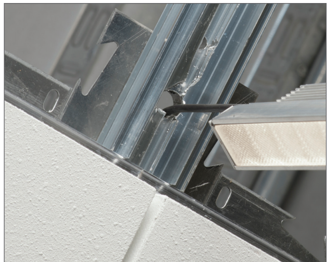
Connection of LED light fixture through Ceilencio ceiling grid
